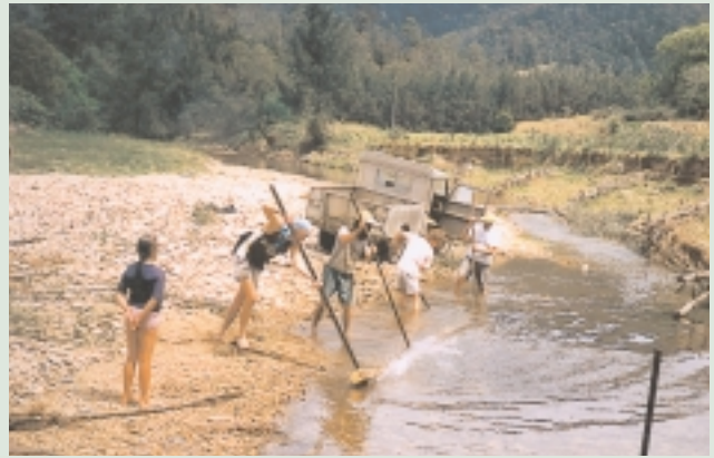
AFTER: The channel was realigned and the group undertook maintenance works.
