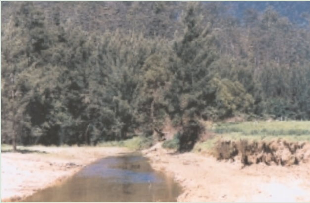
BEFORE: A gravel bench was constructed by the group to widen the channel and stabilise the bank.
